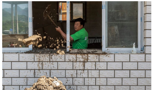
Homestead revitalization - work for relief (road restoration and clean-up)
