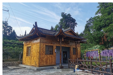
Comfortable Living Environment Program in Yongshun County, Hunan Province - construction of public toilet
