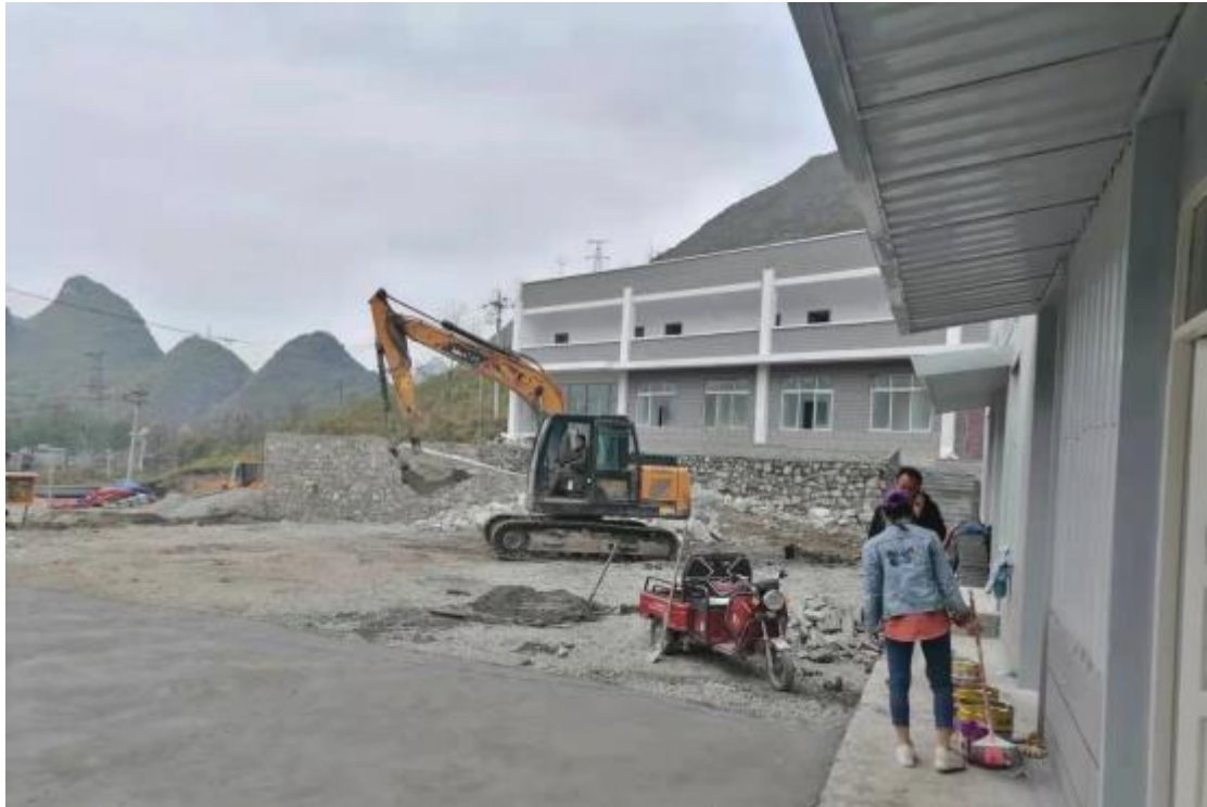
(人才公寓及电商孵化馆周边硬化)
