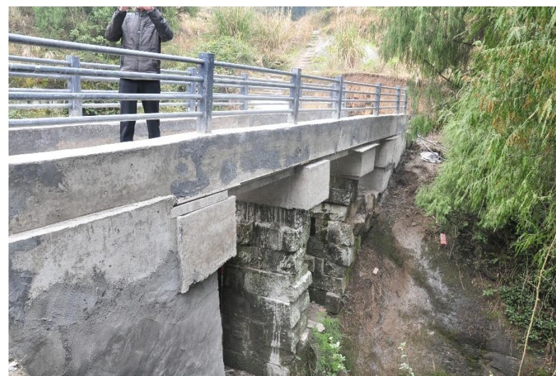
NO.279 堰沟湾过水桥 (已竣工)
